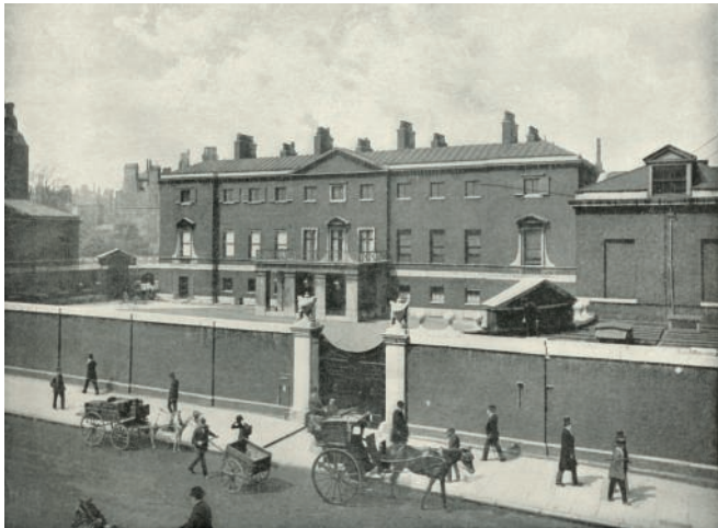
Fig. 1, Devonshire House illustrated for The Queen's London (Cassell, 1896) © Look and Learn / Bridgeman Images
